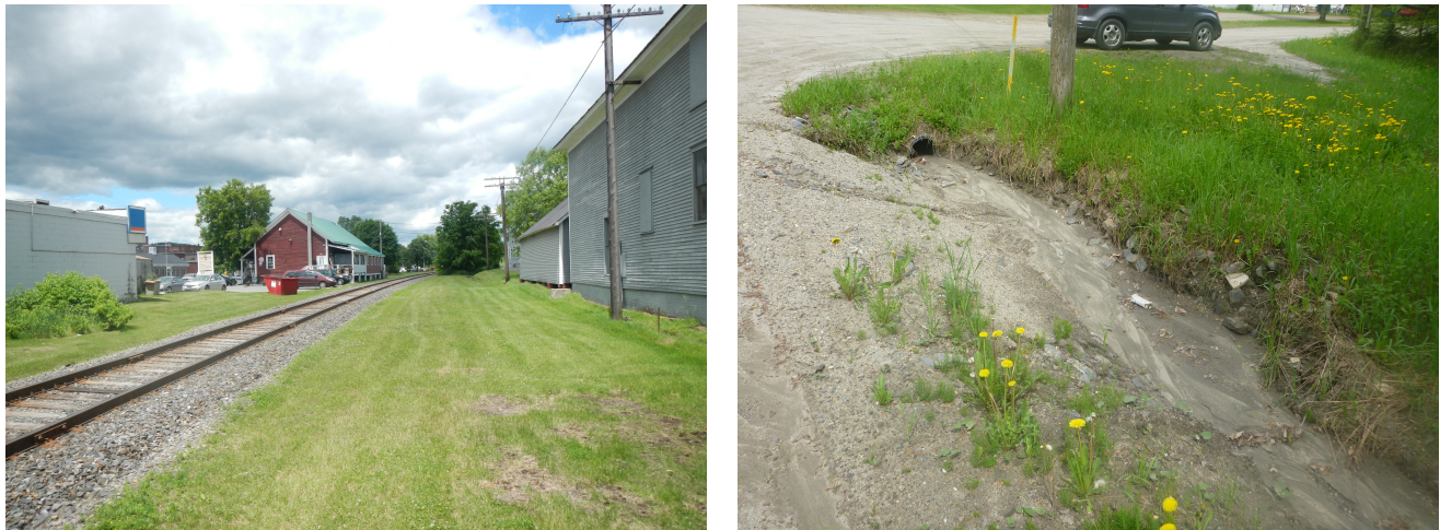
Figure 2: A stormwater pipe carrying runoff from portions of Williams Street to a stable grassed swale infiltration area had the lowest score (Rt5-9). Severe road erosion and large volumes of sediment along Lily Pond Road (LY-8) had the highest problem area score.
