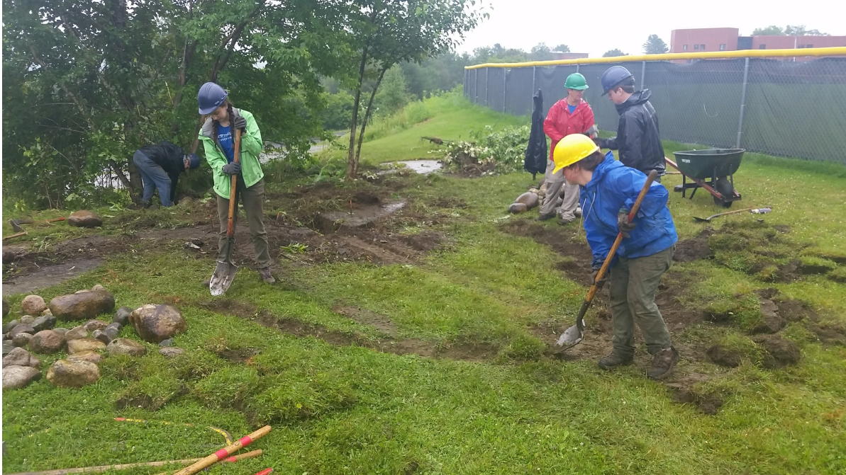
Figure 5: NorthWoods crew beginning site work for the LSC-6 project.
