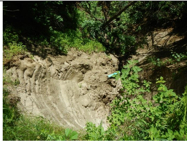
Photo 1: View from the top of the gully.
