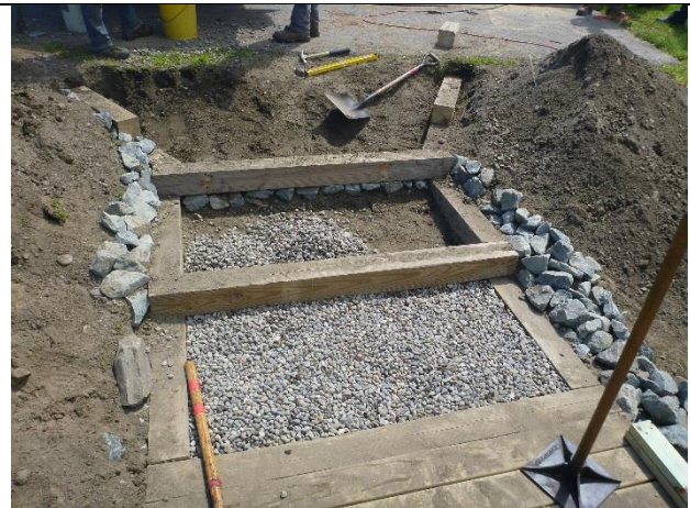
Photo 2: Installation of infiltration steps from parking lot to footbridge.
