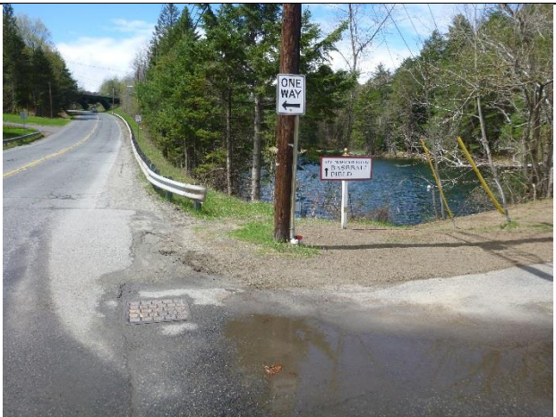
Photo 1: Catchbasin located at the Institute Circle and College Road intersection, drains to the pond.
