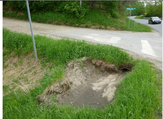
Photo 2: Sediment trap at base of hill in wetland.
