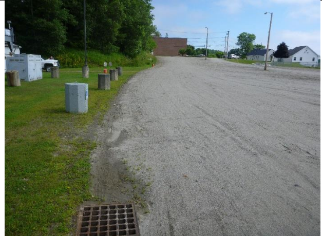
Photo 1: Flow path along the edge of the large gravel parking lot draining into a catchbasin.
