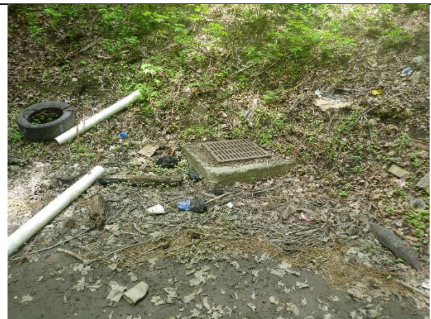
Photo 2: Outlet structure approximately 6" above the basin bottom.
