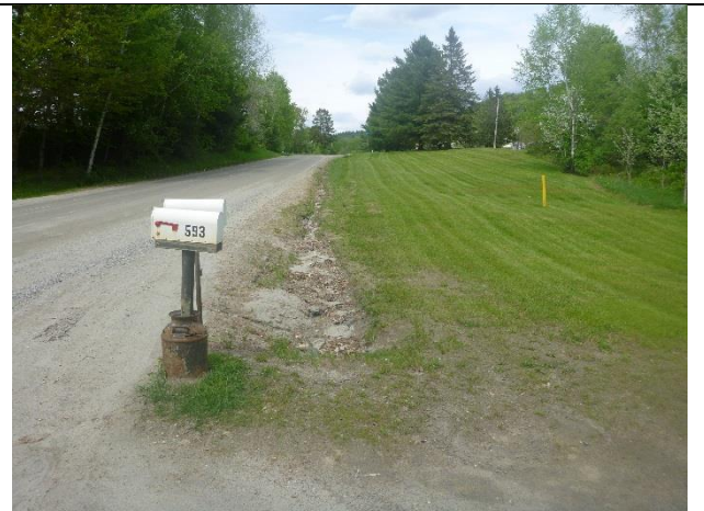
Photo 2: Long ditch section along a moderately steep section of Lily Pond Rd.
