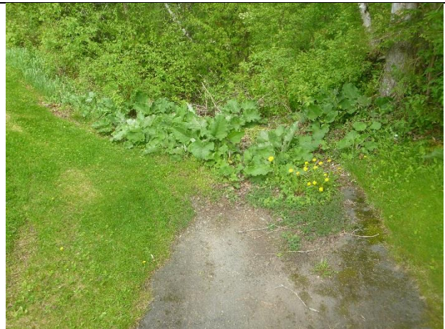
Photo 2: Outlet of ditch to steep forested slope leading to the floodplain.
