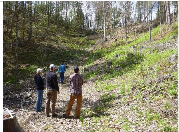
Photo 2: Major erosion along a steep and straight trail section with no stabilization structures.
