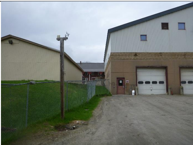
Photo 1: Rooftops draining to catchbasin
