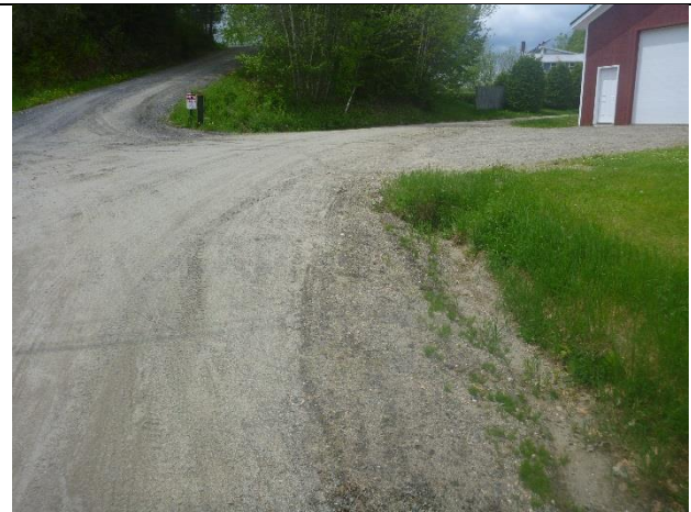
Photo 2: Steep private road and gravel parking draining in to the ditch with rill and gully erosion.
