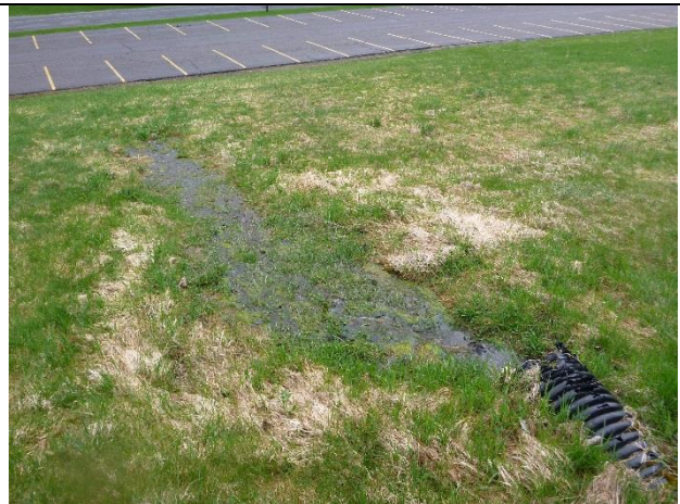
Photo 2: High nutrient runoff from the baseball fields flowing to the site.
