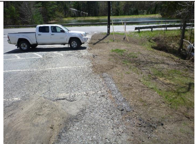
Photo 2: Sheetflow over exposed soil along the steep bank to the pond.
