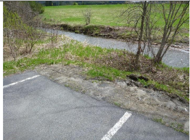
Photo 2: Minor gully erosion along stream bank and exposed soil from plowing.
