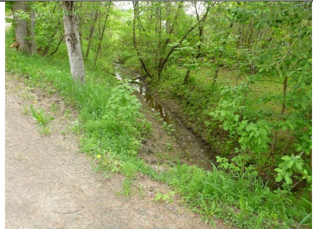
Photo 2: Stormwater cross under road to intermittent stream flowing into a wetland.
