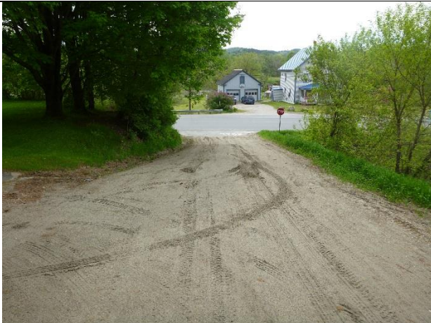
Photo 1: Steep road segment with no ditches, grader berm on south side.
