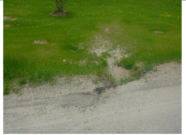
Photo 2: Large gully along road edge with sediment deposits in floodplain.
