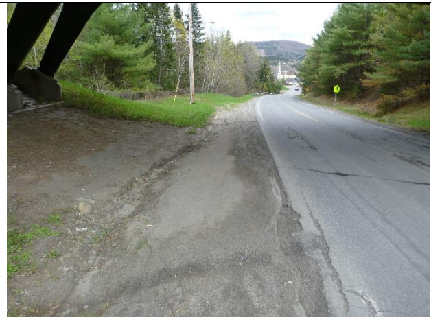
Photo 2: Two eroded flow paths along the road shoulder, some runoff continues down College Rd.
