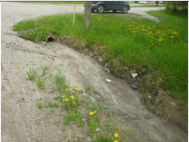
Photo 1: Gully erosion and significant sediment loads in ditch.
