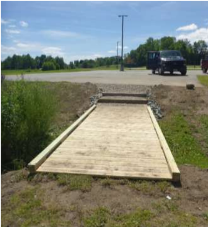
Figure 7: Footpath bridge over the stormwater swale
