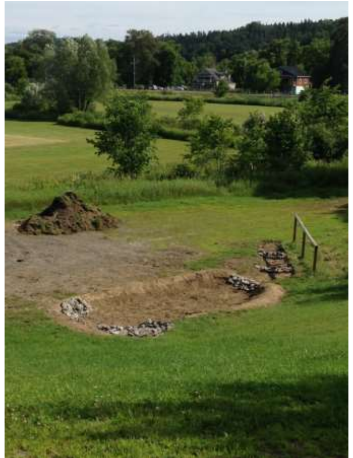
Figure 5: Constructed sediment basin
