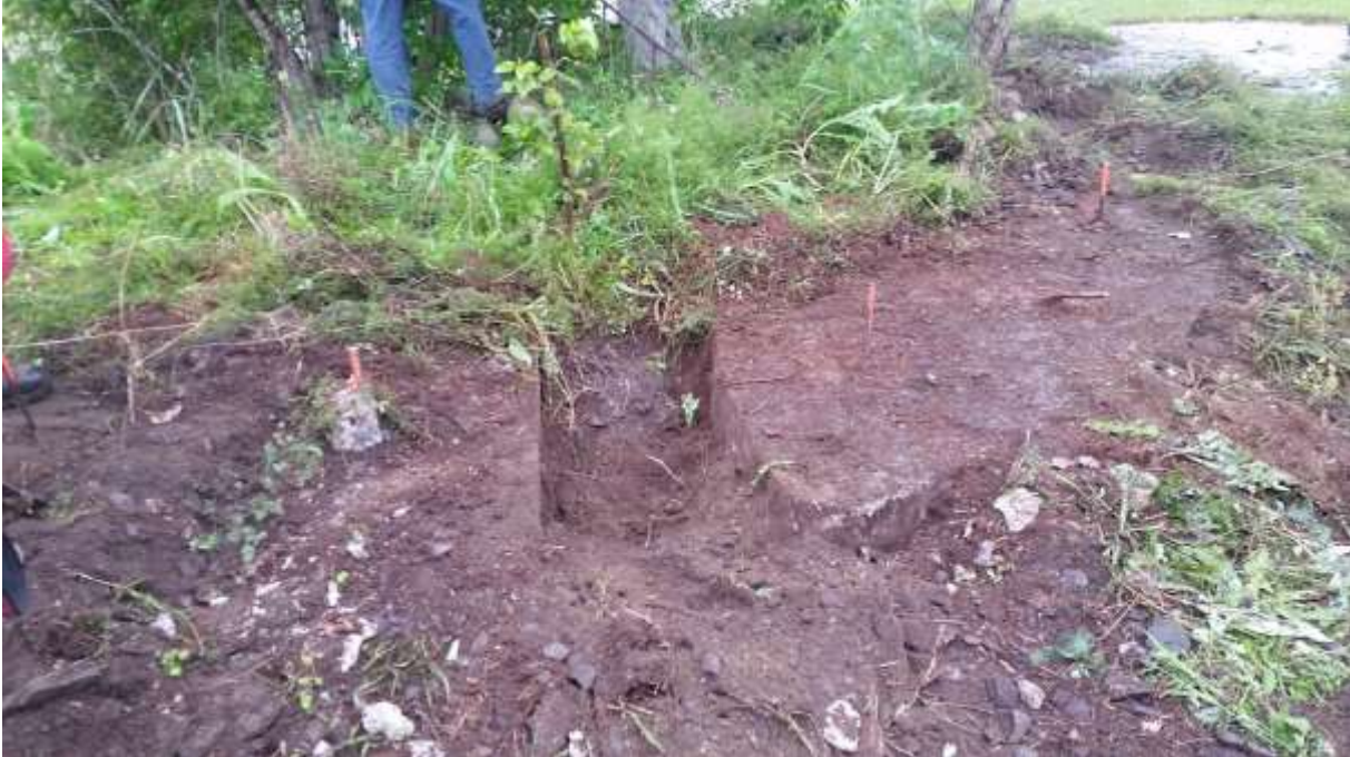
Figure 10: Concrete ring uncovered during excavation
