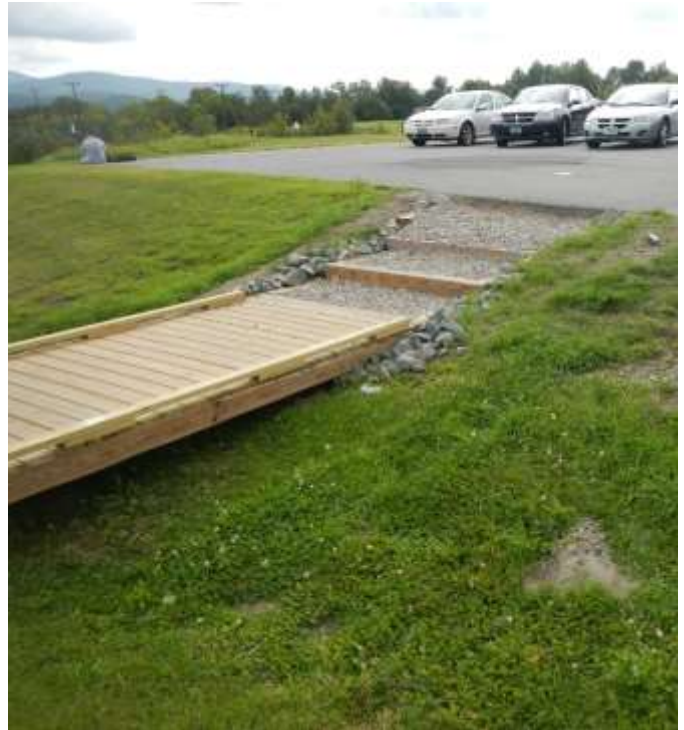
Figure 8: Infiltration steps between the bridge and parking lot
