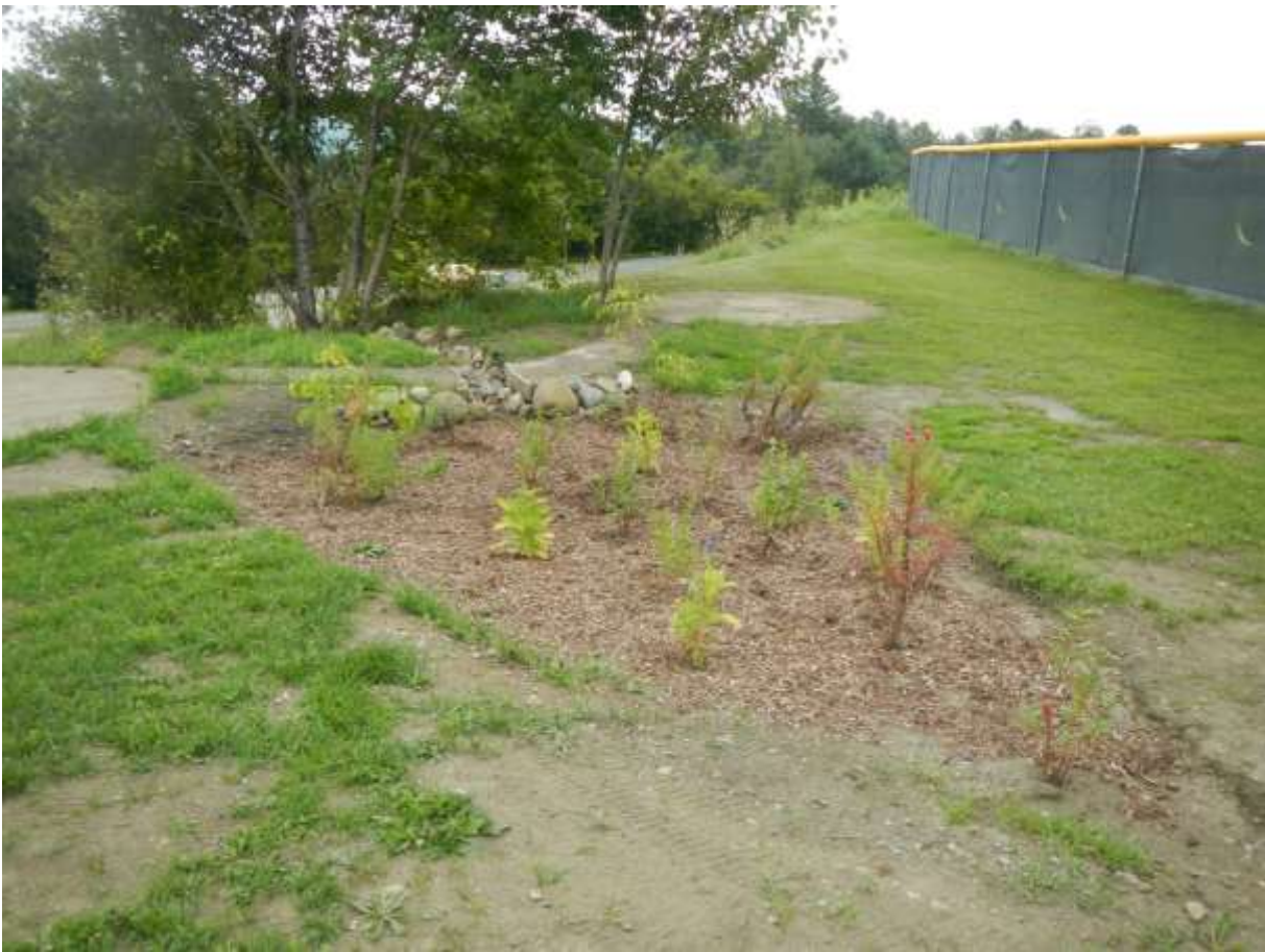
Figure 11: Completed rain garden with some exposed soil from construction disturbance
