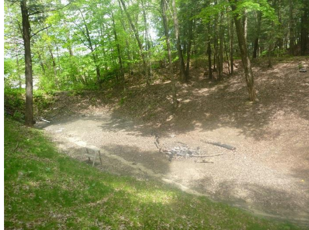
Figure 3: Sediment deposits filling the pond to the outlet structure elevation
