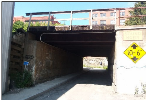
Figure 8: Honking Tunnel, July 2022
