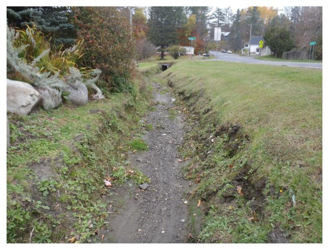
For conceptual design at this site, Stone considered Schumm's Channel Evolution Model (CEM; USDA 2012). The CEM provides a predictable sequence of changes a stream can undergo after disturbances such as channel straightening, increase in peak discharges, or decrease in sediment load (see figure in Appendix D). The changes can include increases or decreases in the
