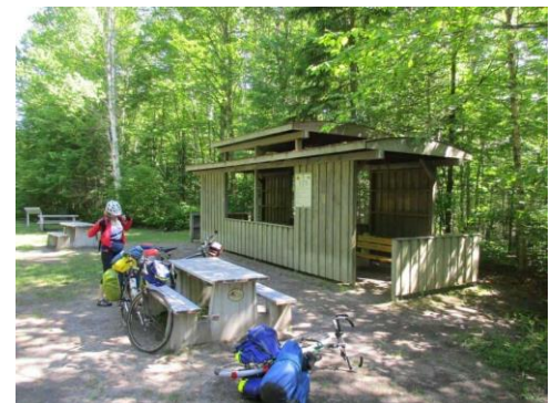
One of the rest shelters along the trail
