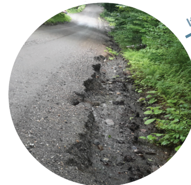
Erosion likely - Unstable Ditch (no rock or grass)
