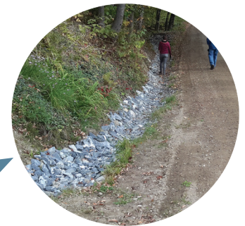
Stone line to prevent erosion
