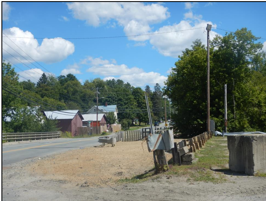
Photo 5. Photo shows the southwest corner at the bridge over the Moose River. View is to the northeast toward structures located on the northeast quadrant of the bridge.
