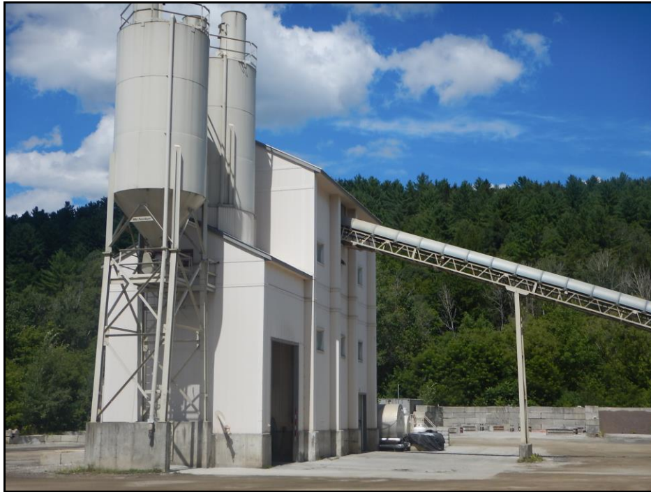
Photo 8. Photo shows the concrete mixing facility located west of the bridge over the Moose River. View is to the north.
