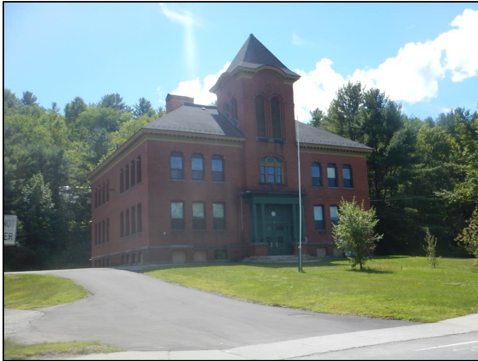
Photo 10. Photo shows the c.1900 Summerville School located on the south side of Portland Street. View is to the south.
