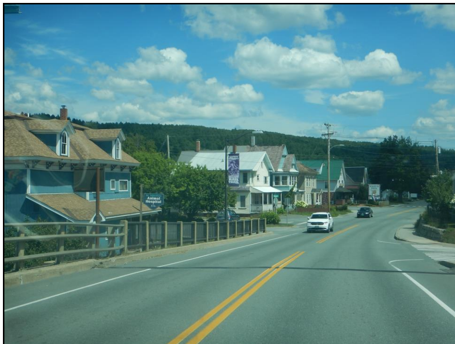
Photo 2. Photo shows the east end of the bridge spanning the Passumpsic River. Note the structures are below the level of the bridge. View is to the east.
