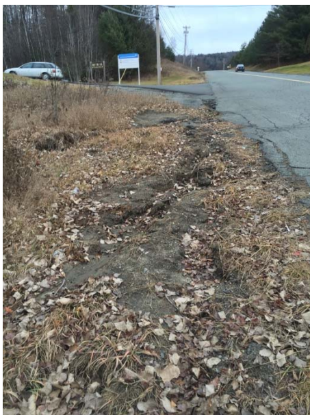
Photo 1: Erosion along the road shoulder
