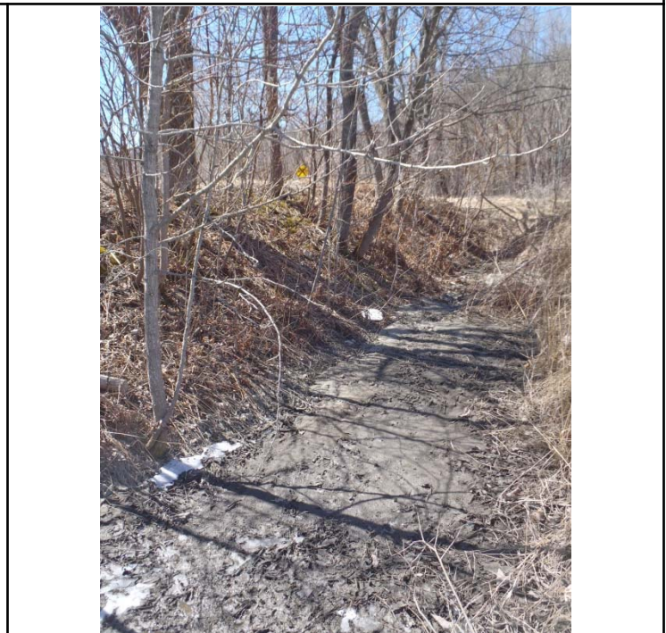
Photo 2. Swale, looking east from Bay St, with sediment deposition
