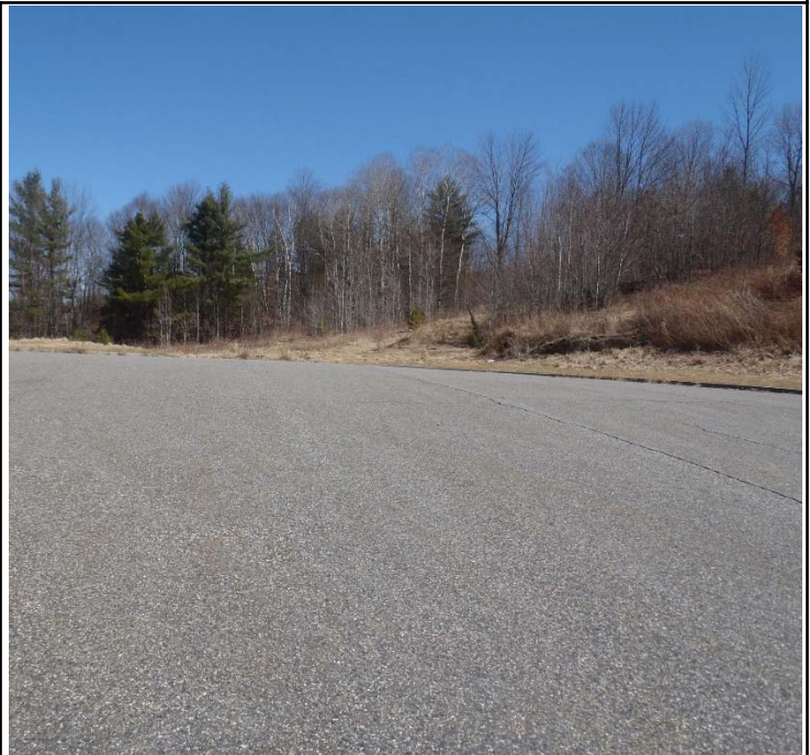
Photo 2. Cul-de-sac at end of Overlook Dr; additional driveways should be encouraged to intersect road with better geometry
