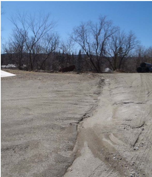
Photo 1. Gully erosion through Town Garage maintenance yard
