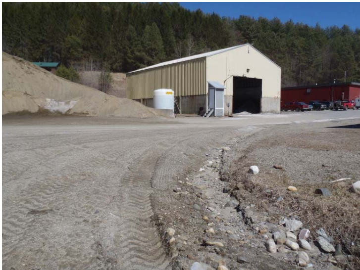
Photo 2. Visible “creep” of the sand storage pile
