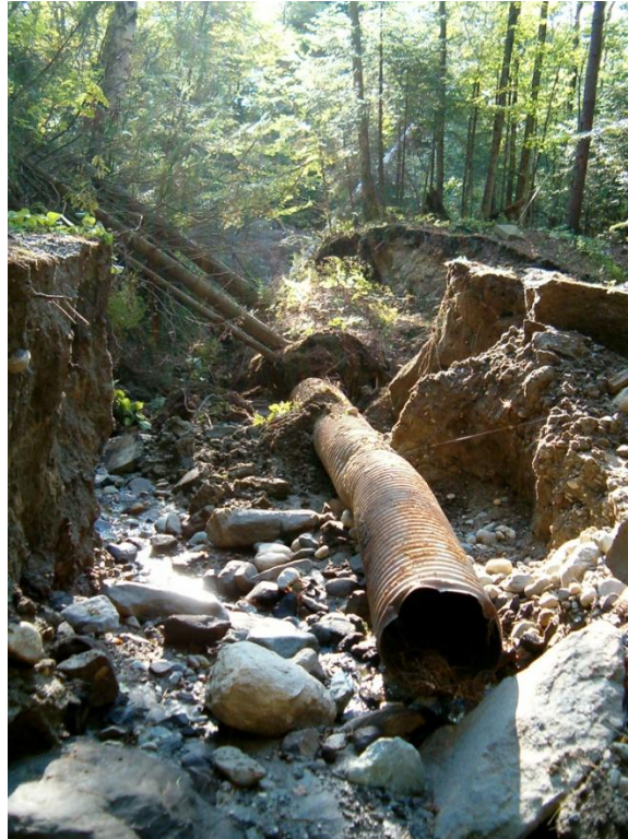
Sand Hill Road – a Class 4 road in Glover after an intense summer rain event June, 2014
