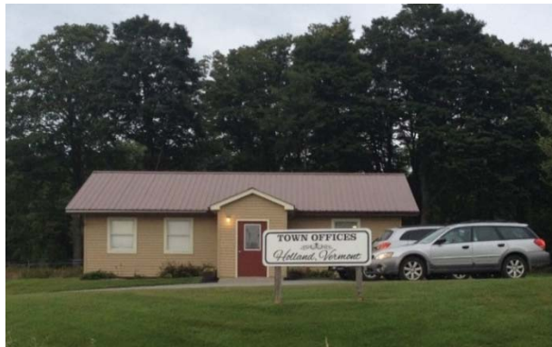
Holland Town Offices
