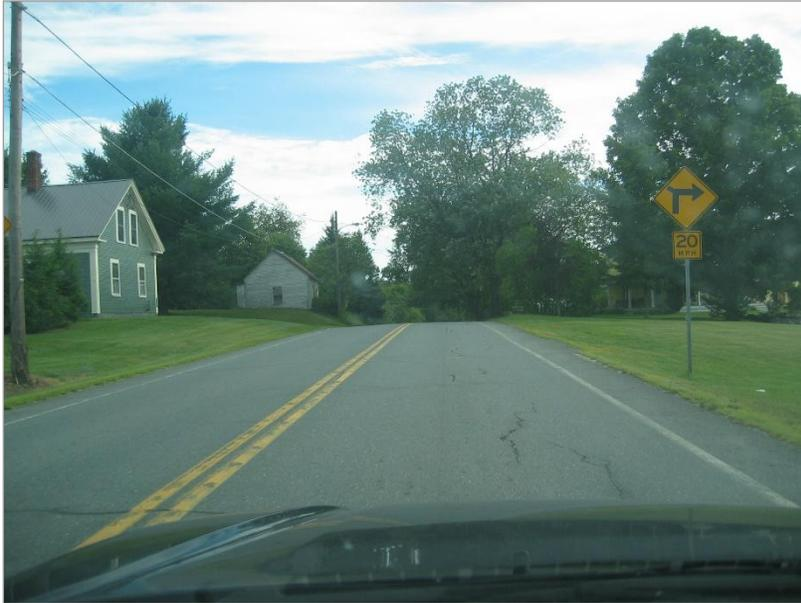
Adequate intersection sight distance (ISD) to the north means vehicles exiting Mountain Road can see far enough along VT 114 to decide whether it is safe to enter VT 114 without colliding with another vehicle. The ISD measured in the field is 150 feet, but it should be at least 200 feet. It would be desirable to have 335 feet of intersection sight distance.
