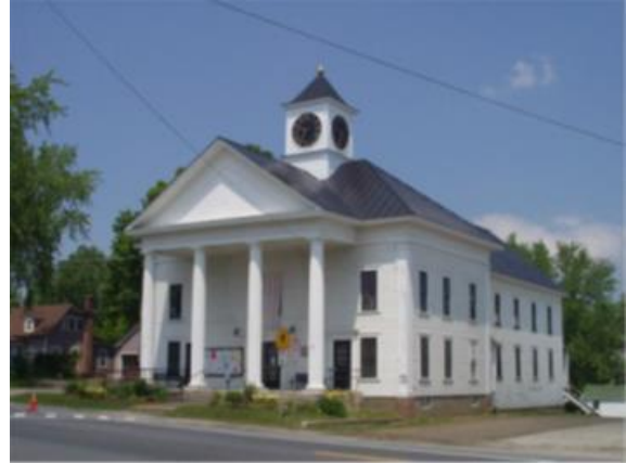
Danville Town Hall and Offices
