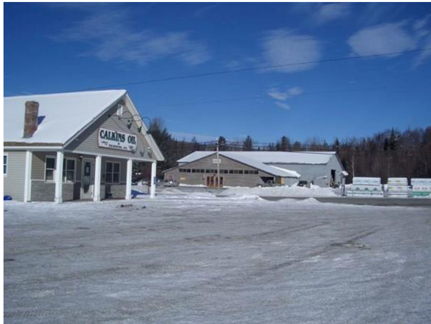
Commercial and Light Industrial Development - Calkins Excavating and Larrabees Building Supply
